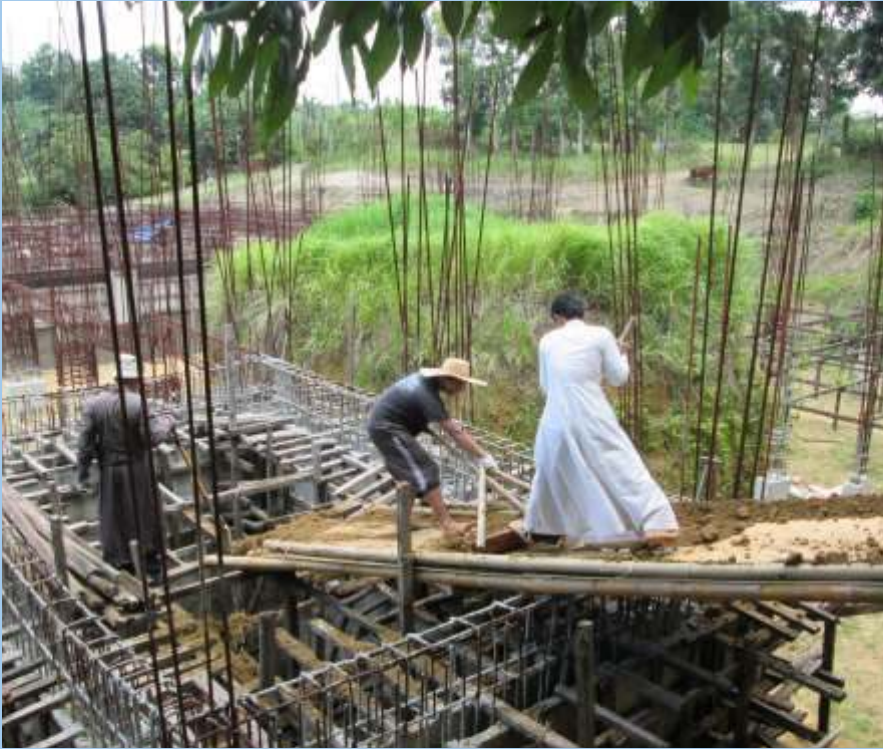
A little African-Philippine engineering! A sand-side constructed to facilitate the refill process. The Brothers seem to find their second childhood on this side!!
