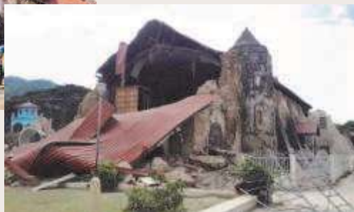
Tragedy: the intricately-designed facade of the 18th century Church of San Pedro Apostol in Loboc, Bohol completely collapsed in the earthquake of October 15th 2013. ....
